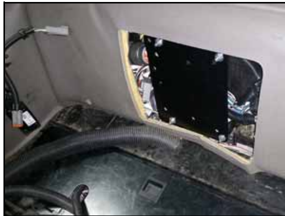
FIGURE 8. HDU Mounting Bracket Installed
