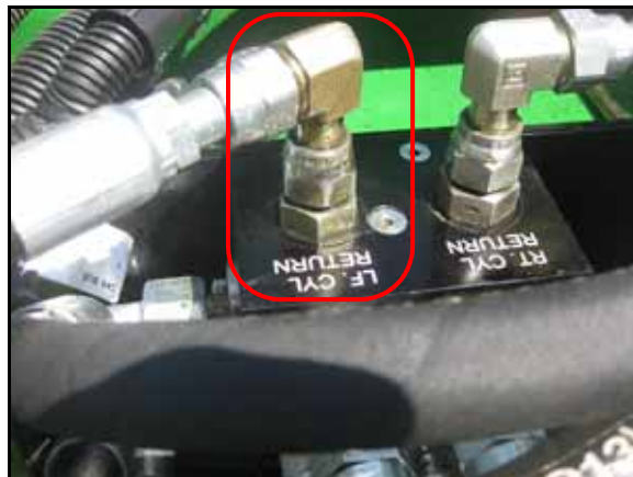
FIGURE 24. Left Down Hose Installed on AutoBoom Valve
