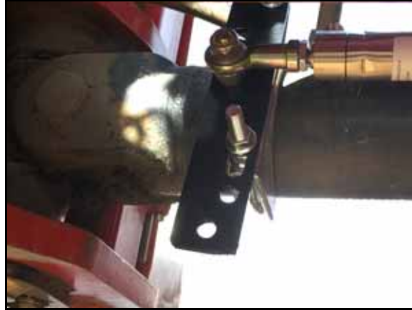
FIGURE 10. Base-End of WAS Installed
