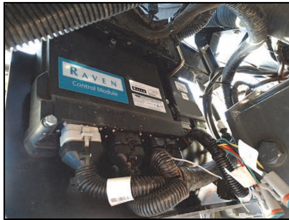
FIGURE 5. AutoBoom Cable Connected to Node
