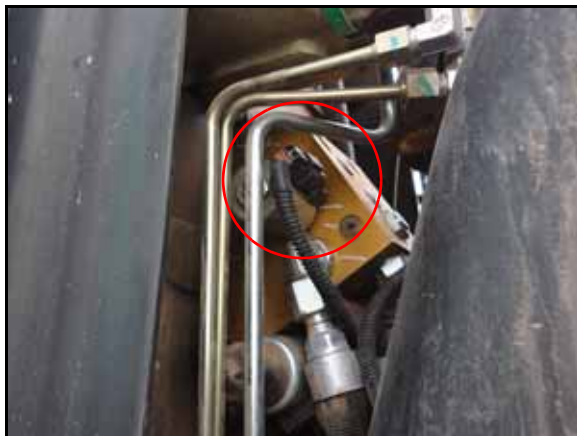
FIGURE 9. ISOLATION Connector Installed on Valve
