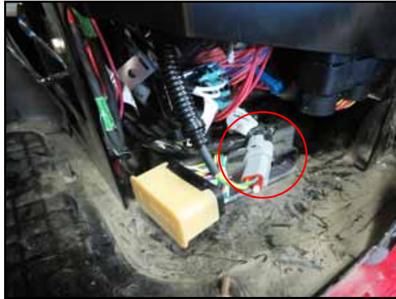
FIGURE 9. 3-Pin Deutsch Connected to Terminator Location
