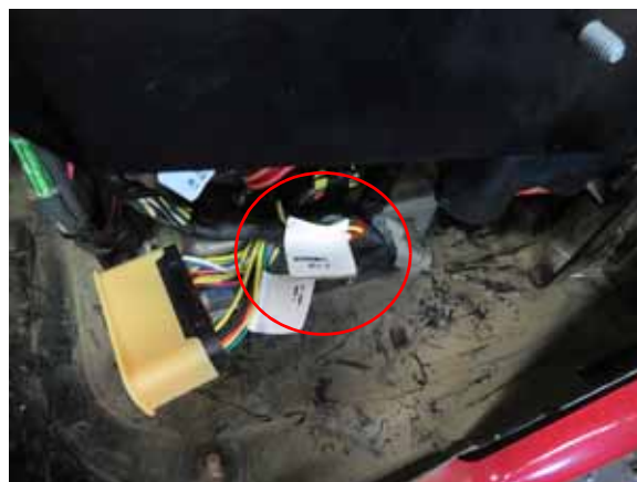
FIGURE 8. 12-Pin Deutsch Installed Near Steering Connectors
