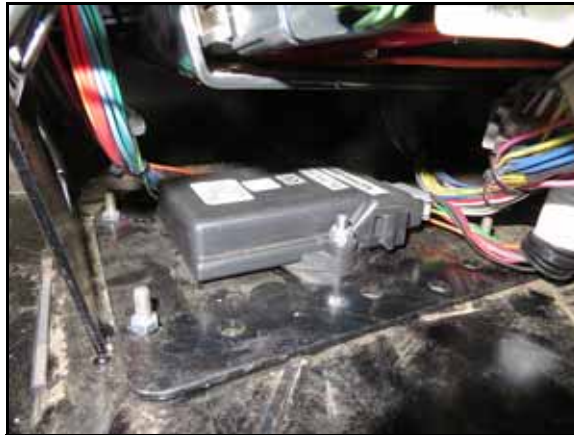
FIGURE 3. Node and Bracket Secured to Floor Studs
