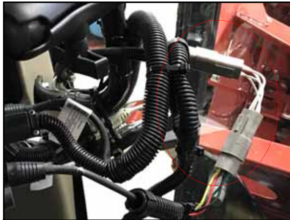
FIGURE 9. CAN Bridge Cable Connected to SC1/HDU Harness Cable
