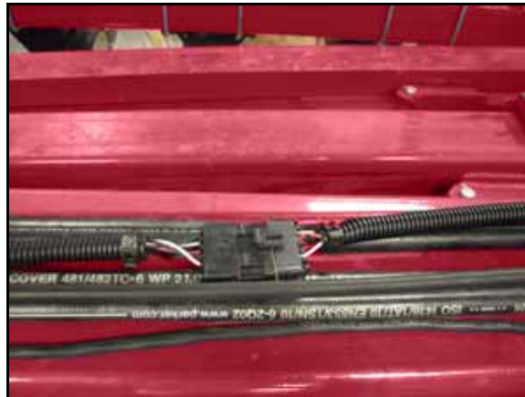
FIGURE 3. Harness Cable and Adapter Cable Connection
