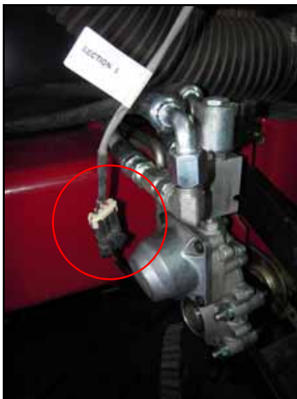
FIGURE 4. Harness Cable Connections on the Row Units
