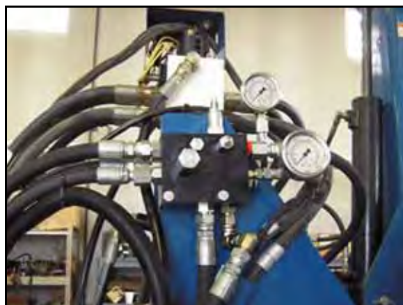
FIGURE 18. Pressure-Reducing Valve Pressure and Tank Hoses Installed
