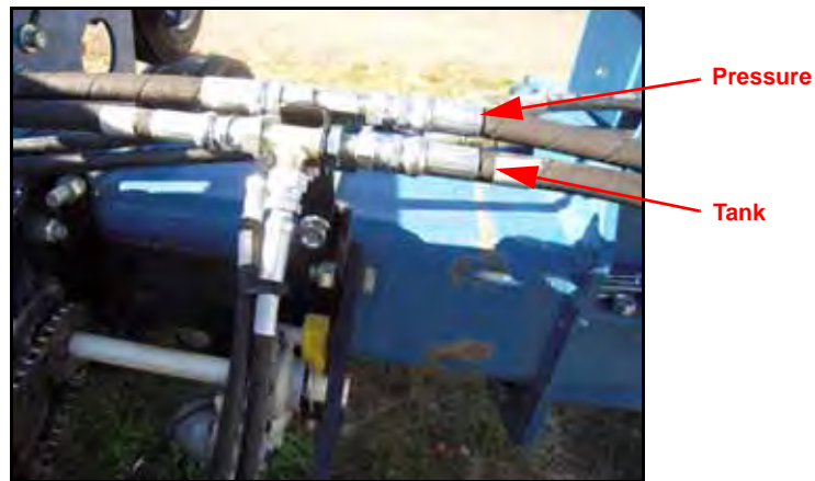
FIGURE 17. Planter Row Unit Pressure and Tank Hoses Installed
