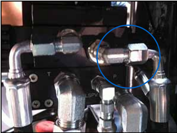
FIGURE 10. Right Steering Hose Installed on Steering Valve
