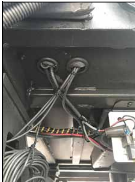
FIGURE 20. Feeding HDU Cable out of Cab
