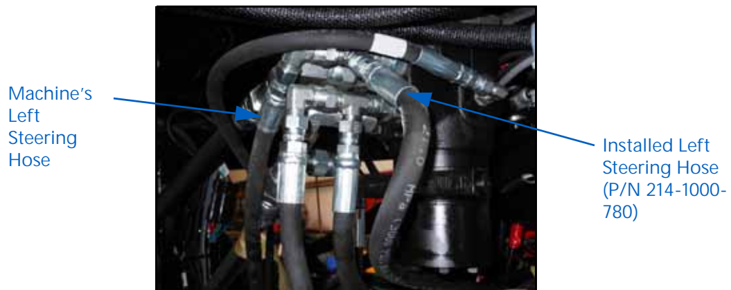
FIGURE 6. Left Steering Hose Installed on Steering Orbital
