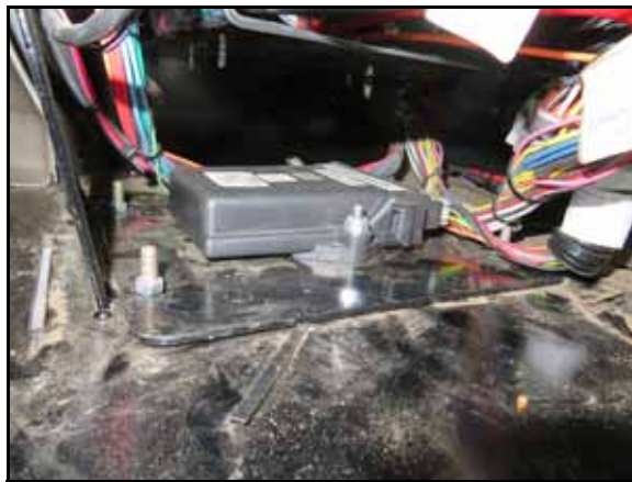
FIGURE 15. ECU Harness Installed on ECU
