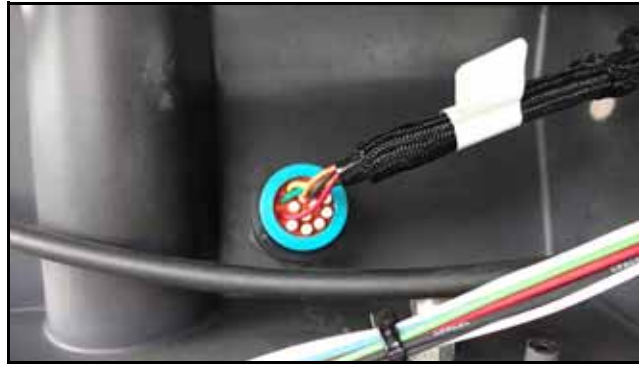
FIGURE 3. Completed Bulkhead Connection
