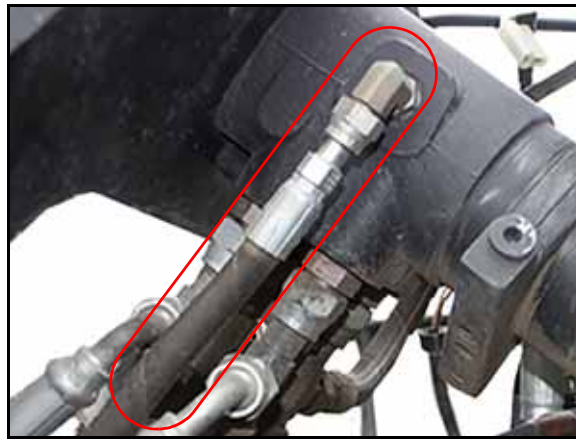
FIGURE 11. Load Sense Hose Installed on Steering Orbital
