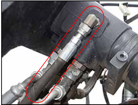
FIGURE 11. Load Sense Hose Installed on Steering Orbital
