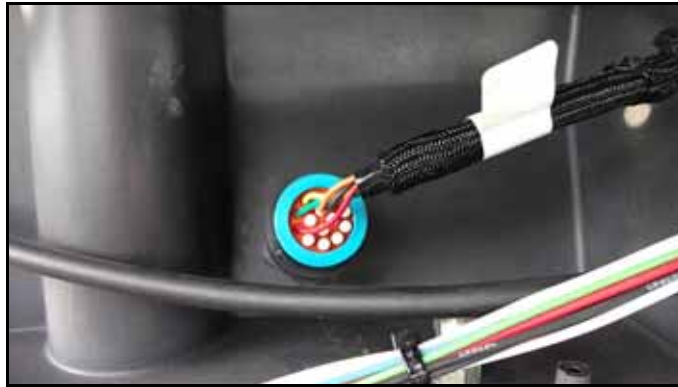
FIGURE 3. Completed Bulkhead Connection
