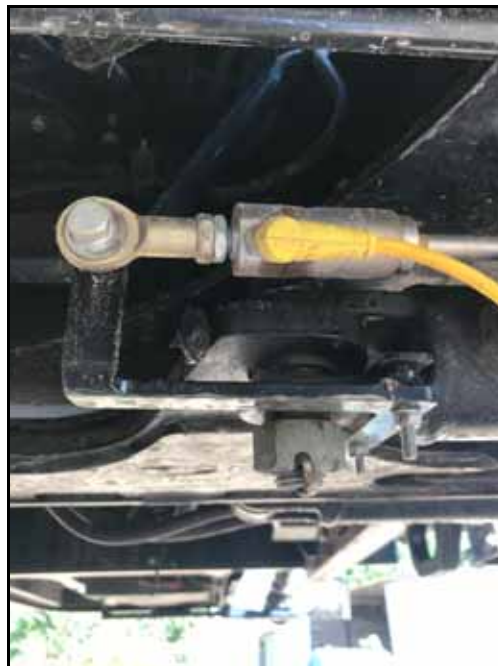
FIGURE 2. WAS Base End Mounting Brackets Installed
