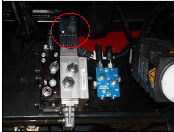
FIGURE 19. Valve Harness Cable Installation Location
