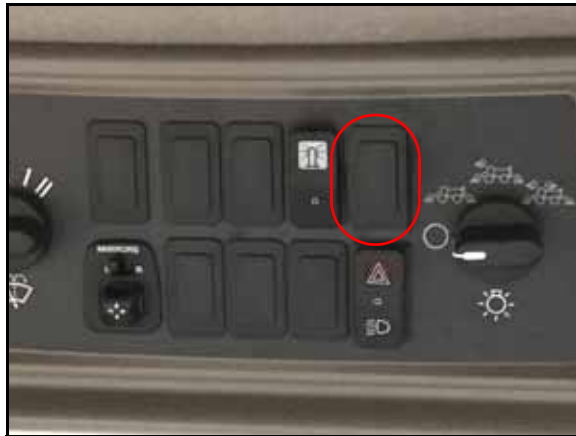
FIGURE 14. Master Switch Installation Location
