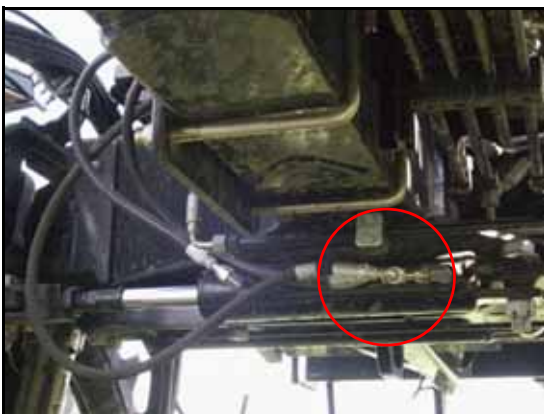
FIGURE 9. Installed Right Steering Hose
