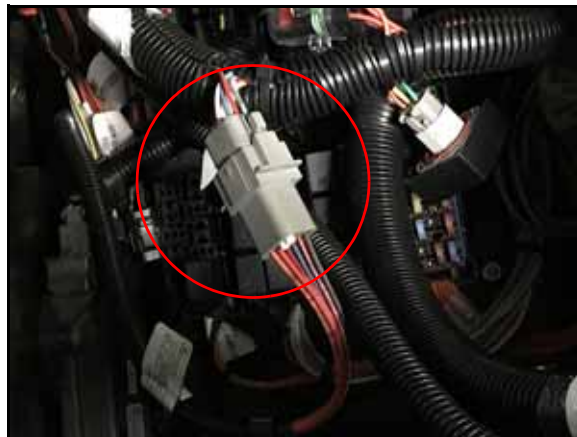
FIGURE 12. HDU Harness Cable Connection
