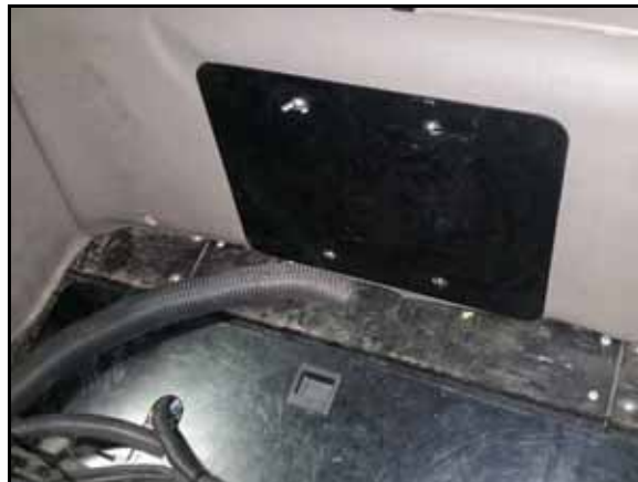
FIGURE 4. Access Panel to be Removed
