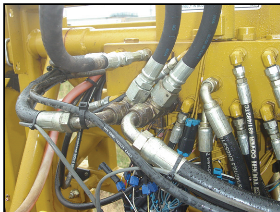
FIGURE 4. Left and Right Cylinder Hoses Installed
