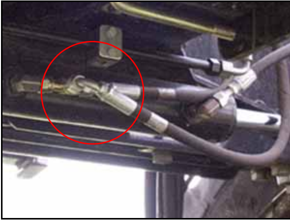
FIGURE 8. Installed Left Steering Hose
