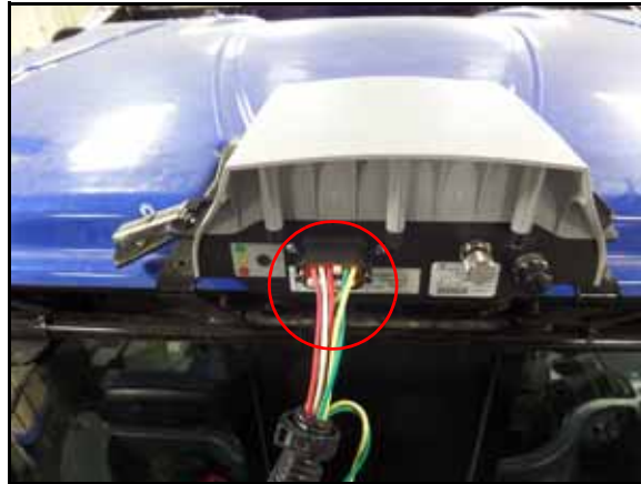
FIGURE 7. RS1 Harness Installed on RS1 Unit
