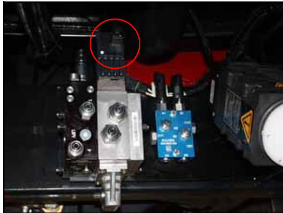
FIGURE 18. VALVE Harness Cable Installation Location
