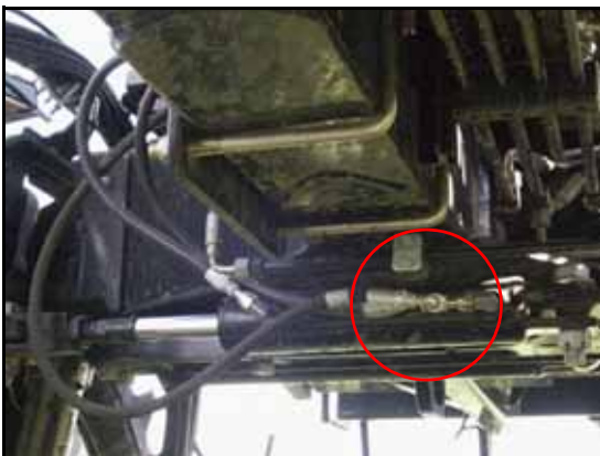
FIGURE 9. Installed Right Steering Hose on Left Steering Cylinder
