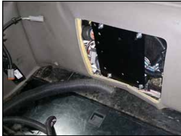
FIGURE 16. HDU Mounting Bracket Installed
