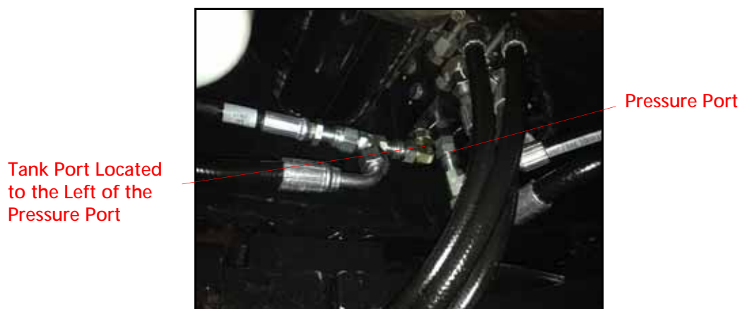
FIGURE 7. Tank Hose Installed
