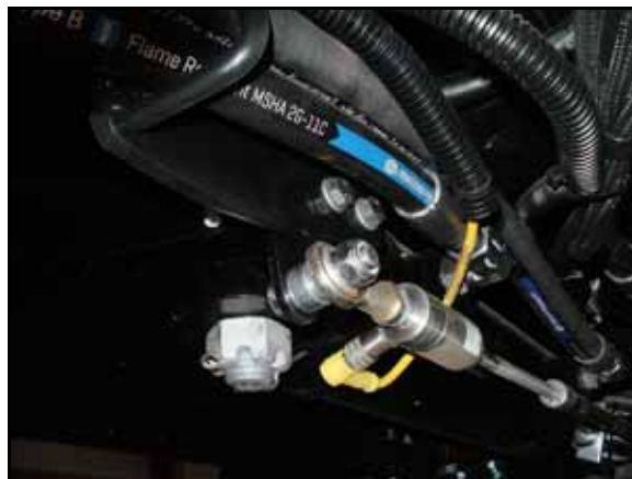
FIGURE 6. WAS Adapter Cable Installation
