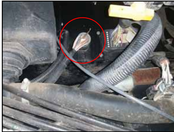
FIGURE 13. RS1 Tee Cable Connected to Machine's Bulkhead
