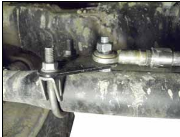
FIGURE 10. Rod End of the WAS Secured to the WAS Bracket
