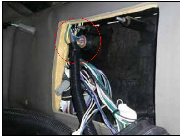
FIGURE 5. Machine's XB-7 Bulkhead Connection
