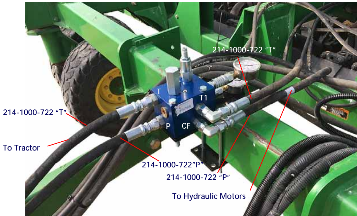
FIGURE 22. Hoses Connected on Manifold
