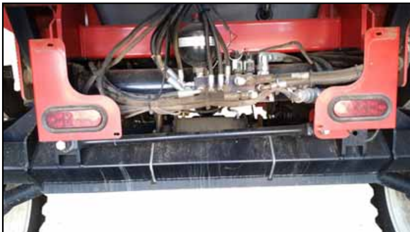
FIGURE 1. Hoses Routes Beneath the Structural Cross Member
