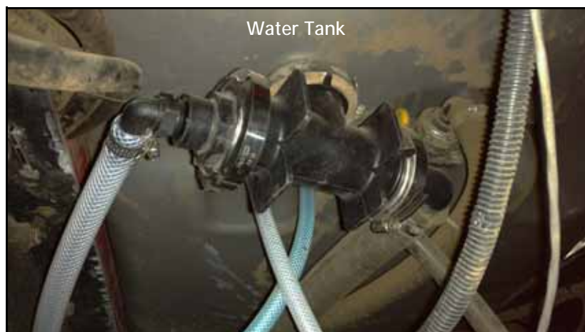
FIGURE 13. Completed Tank Tee Installation
