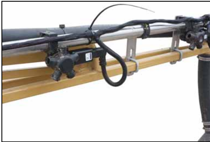
FIGURE 13. Securing Valve Branches
