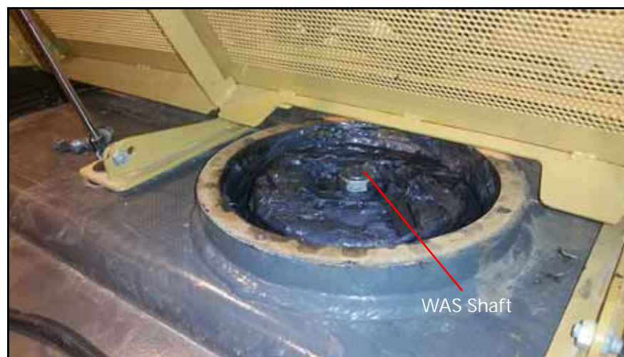
FIGURE 21. Installed WAS Shaft
