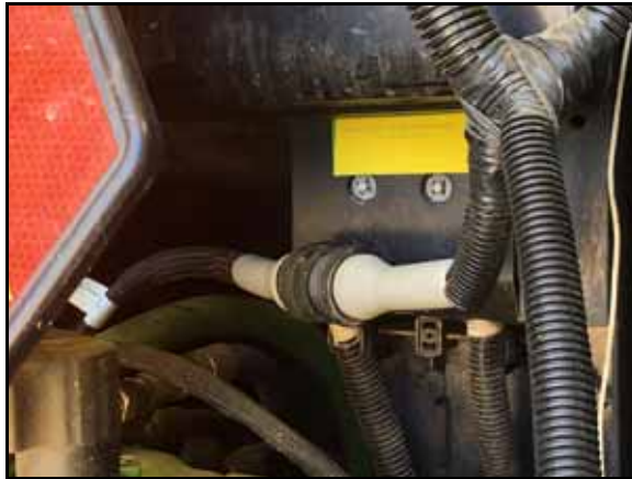
FIGURE 9. 15' RS1 Tee Cable Connected to Machine's Power Cable
