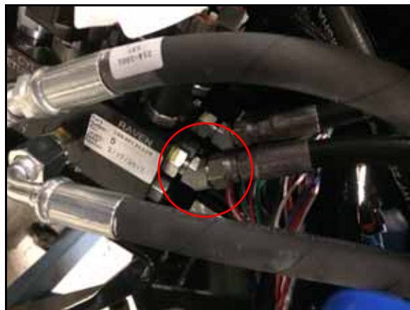
FIGURE 7. Left Cylinder Hose Installed on AutoBoom Valve
