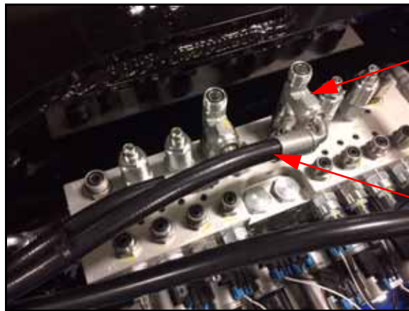
FIGURE 6. Left Cylinder Hose Installed on Machine's Hydraulic Valve
