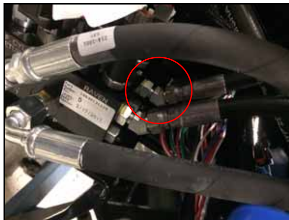
FIGURE 9. Right Cylinder Hose Installed on AutoBoom Valve
