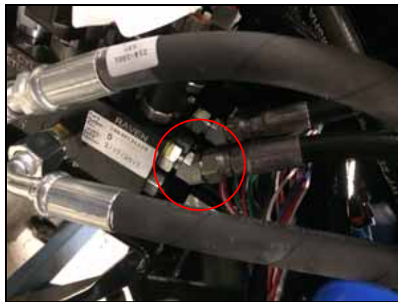
FIGURE 7. Left Cylinder Hose Installed on AutoBoom Valve
