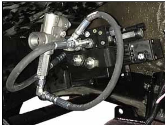
FIGURE 3. Hoses Installed on SmarTrax and Load Sense Priority Valves
