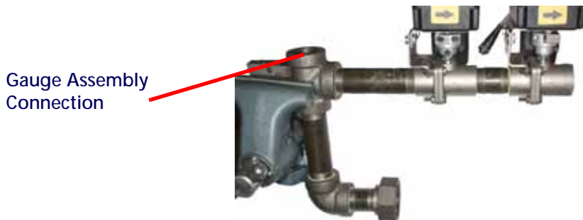
FIGURE 11. Gauge Assembly Connection Location
