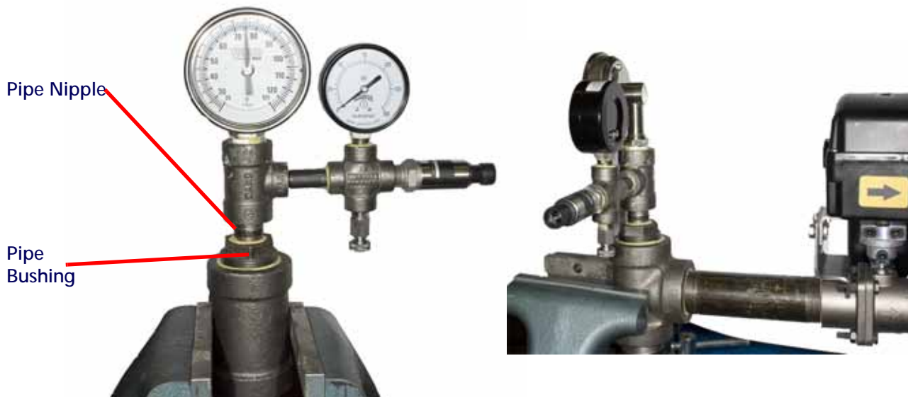
FIGURE 12. Plumbing the Gauge Assembly
