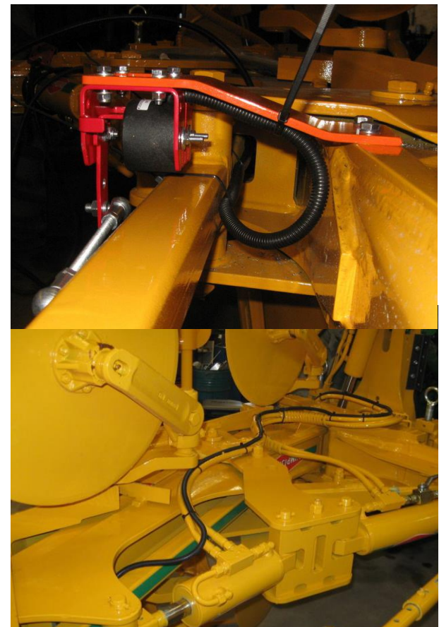
Figure 11 Installing angle sensor lead alongside the hydraulic lines
