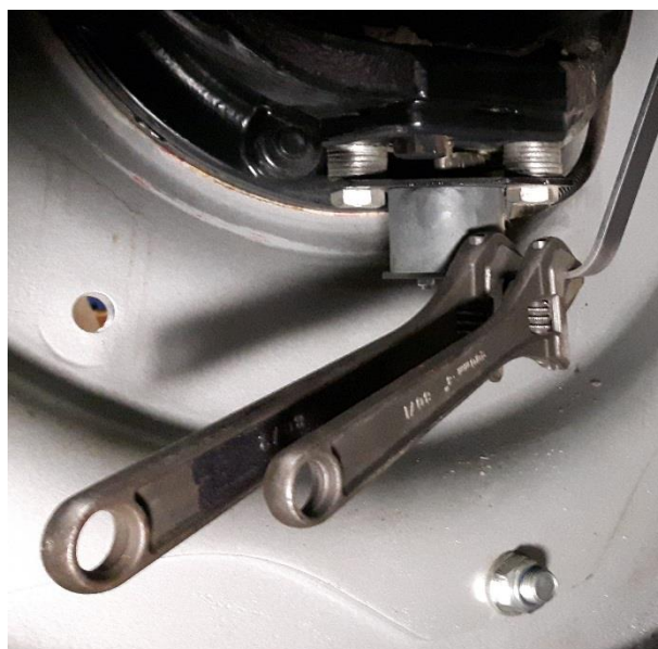
FIGURE 13 BEND THE STRIP WITH THE HELP OF TWO BAHCO'S.
