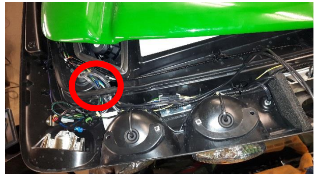
FIGURE 18: CABIN ROOF, PLACE TO GO INSIDE THE CABIN AT THE RED CIRCLE
