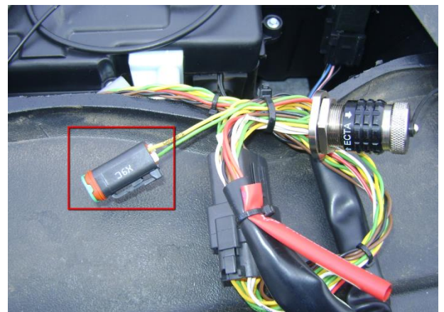
Figure 6 CAN connection on the roof
