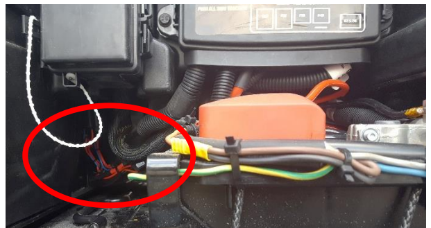
Figure 3 mounted relays and fuses
